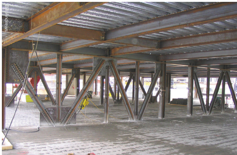
Story-height transfer trusses are enclosed in residential unit partition walls. Including a Vierendeel panel at midspan allows a corridor to pass through the truss.
