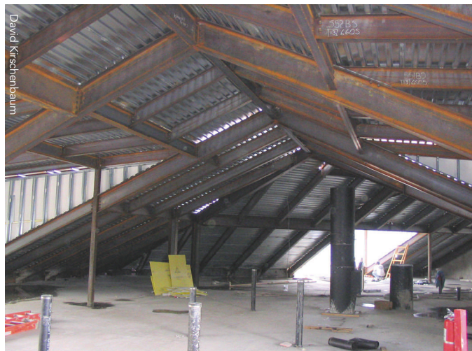
Steel framing sloped to varying pitches supports heavy snow drift loads while also providing usable attic space.
